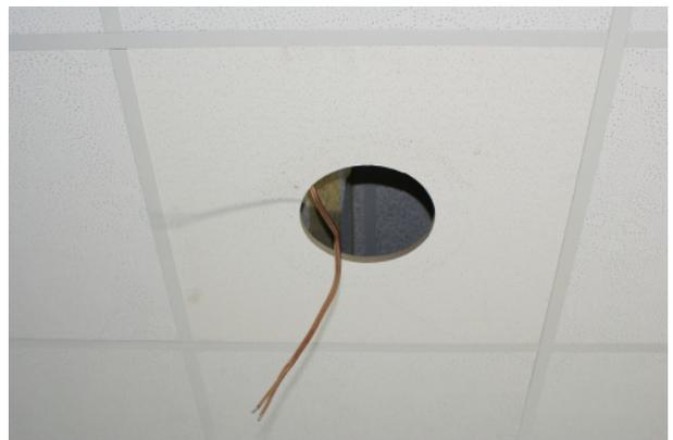
8.) Connect the loudspeaker cables to the jacks of the In-Ceiling loudspeaker that are on the rear side of the speaker. The correct polarity is important here (marked wire = positive pole, must be connected to red terminal, negative pole = must be connected to black terminal). Press on the terminal and insert the cables through the hole on the side of the terminal and release the terminal again.
