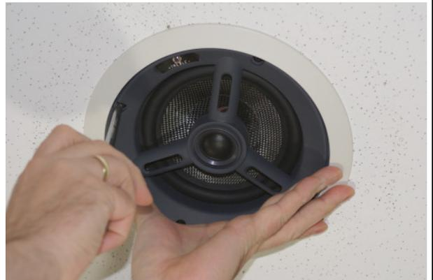
10.) In some cases it might be useful to adjust the tweeter to the listening position. Because the tweeter is pivot mounted, it is possible to adjust it in a wide range. Use your finger tip to adjust the tweeter angle by pressing the outer contour of the tweeter. Be careful not to touch the tweeter's dome.
